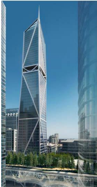
Figure 1 | Southwest Elevation View (Courtesy of Heller Manus)
